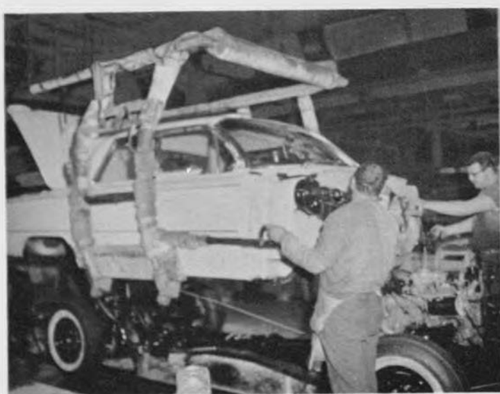
INDUSTRIAL PROGRESS—1961: A far cry from the Linden-made trolley cars of 1907, automobiles by the thousands roll off the assembly lines of the General Motors plant—typical of the industrial productivity of Linden's 146 factories, plants and shops. In this view body and chassis come together at an important point on the assembly line.
